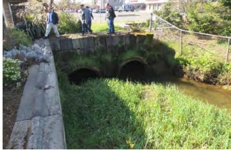
Culvert Constrictions
