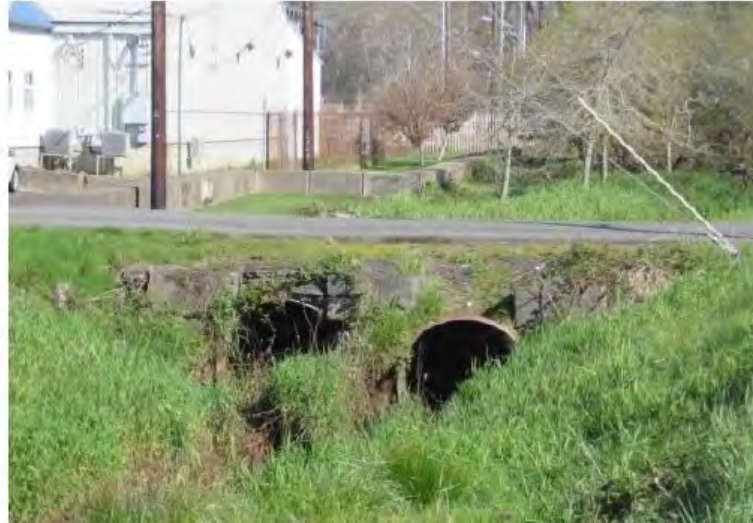
Culvert Constrictions
