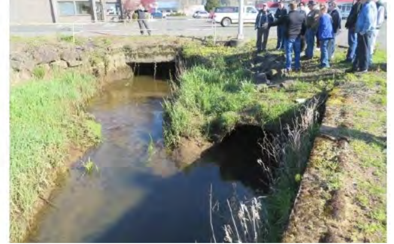
Culvert Constrictions
