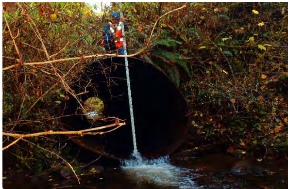
Fish passage barrier corrections opening up 100+ miles of salmon and steelhead
